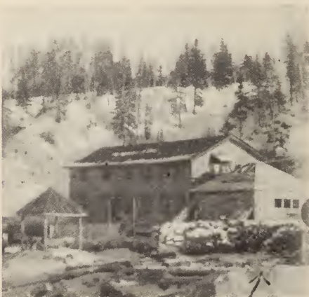
The Mission House with the new laundry at the right
